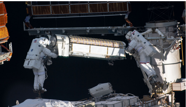
Astronauts Shane Kimbrough and Thomas Pesquet installing the new ISS Roll-Out Solar Arrays (iROSA). (NASA photo)
