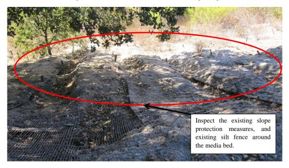
Figure 7: B-1 Media Filter Recommendation 2 (Looking from the B-1 media filter up the adjacent slope)
