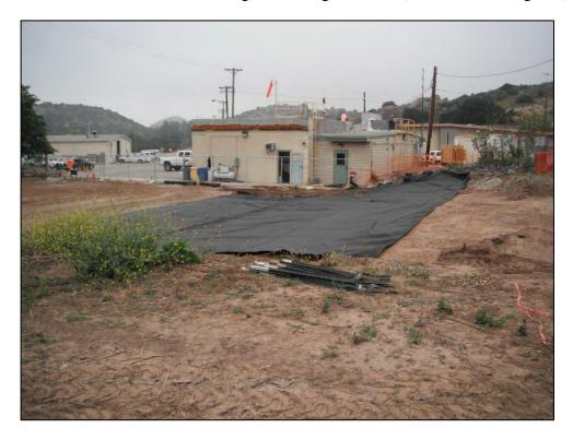
View of ISRA area IEL-2 during liner placement over gravel backfill (6/7/2011, looking east).
