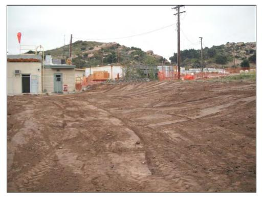
View of ISRA area IEL-2 after soil placement over liner and re-contouring (6/8/2011, looking east).
