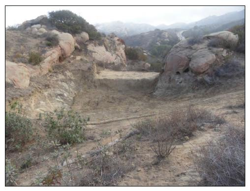
View of ISRA area ELV-1D excavation after contouring and installation of jute matting and fiber rolls (11/20/2013, looking east).
