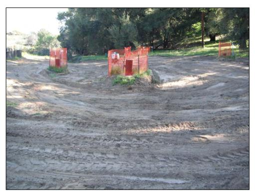
View of ISRA area AP/STP-1E-2 after soil contouring and prior to hydroseed application (2/28/2013, looking east).
