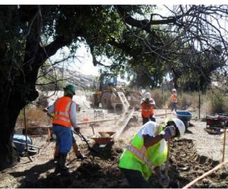
• Soils were removed from the excavation area by wheelbarrow and conveyor belt
