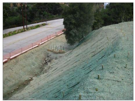
Figure 4. View of lower portion of B1-2, subsequent to ISRA activities. Photograph is toward the northeast, taken on February 17, 2011. Slopes are covered in jute netting and are hydroseeded.
