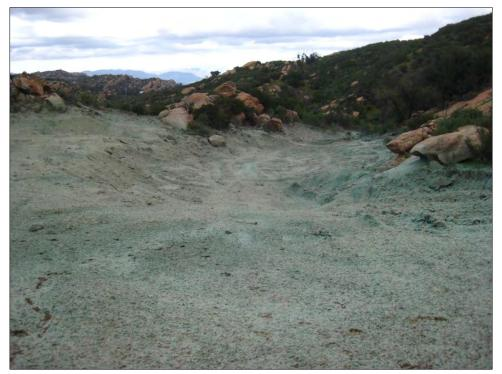
Figure 10.View of Soil Borrow Area, subsequent to ISRA activities, including hydroseeding. Photograph is toward the east, taken on February 17, 2011.
