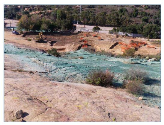
ISRA area B1-2 in background during excavation, ISRA area B1-1B in foreground after restoration with green-blue hydroseed mulch visible (11/19/2010, looking northwest). Orange fencing around Santa Susana tar plants and monitoring wells.
