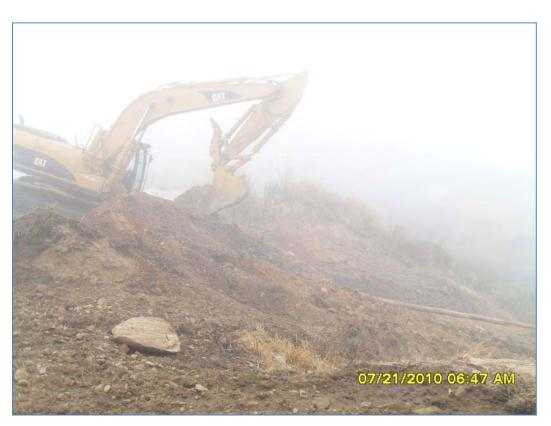
ISRA area CTLI-1A during excavation (7/21/2010, looking west). Previously buried pipeline segment is visible and was subsequently removed (see Appendix H for details).
