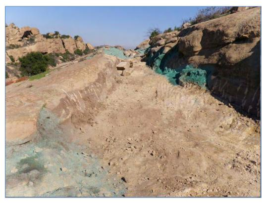
ISRA area B1-1D, west leg, after restoration (11/16/2010, looking northeast). Blue-green hydroseed mulch is visible, bedrock present where hydroseed mulch not applied.
