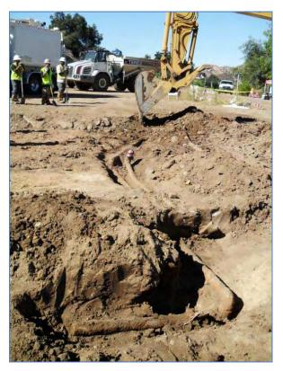
ISRA area B1-2 during excavation (9/17/2010, looking southwest). Encountered buried pipeline visible. Several buried pipelines encountered within the excavation boundary were removed (see Appendix H for details).
