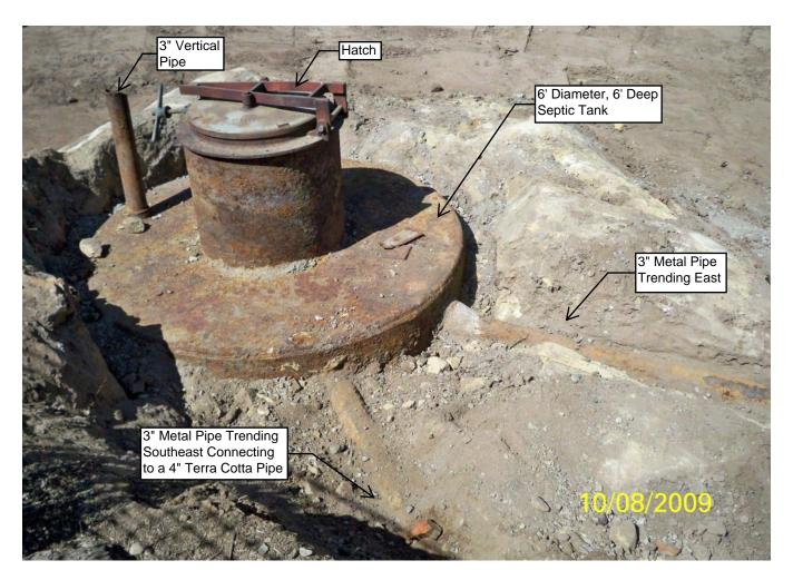
2009 Photograph of the Septic Tank and Associated Piping, Looking North
