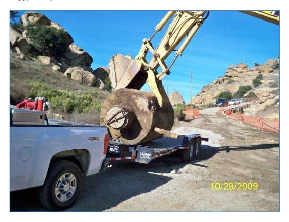
View of septic tank being loaded onto a flatbed truck for transport offsite, Happy Valley South, 10-29-08.
